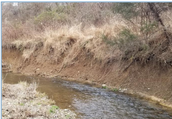
Prior to restoration, banks within this stretch of stream were heavily eroded, measuring 5+ ft. high in some areas.
